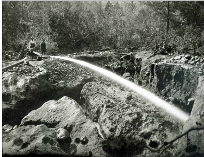
Figure 9. Hydraulic mining in the Etowah Watershed.
